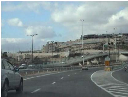
Israeli route: By-pass road A60 North.
