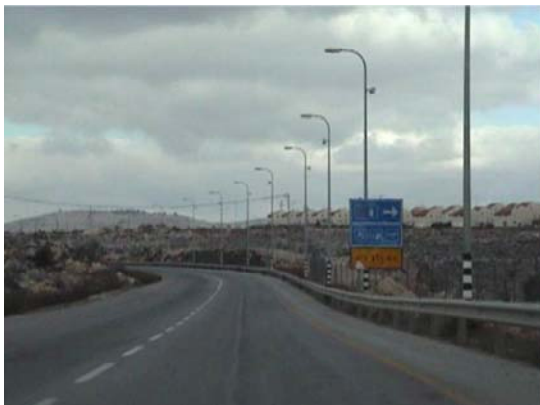
Israeli route: By-pass road A60 North near the colony.
